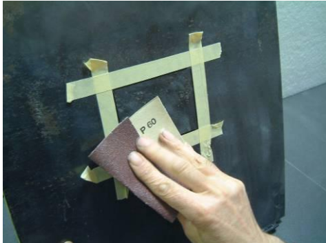
3. Abrade the substrate area to be glued
