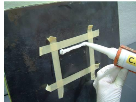
6. Applying C.TAG/® UW2 adhesive from the cartridge Nozzle ends should be cut to allow a proportionate amount of adhesive to be applied to the prepared substrate area.
