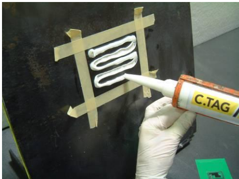
7. Once the adhesive is dispensed .....
